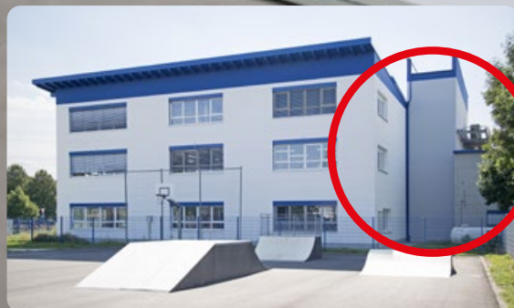
Extensive tool warehouse with three towers of 12 meters height and customized widths in the interspace of two production halls
